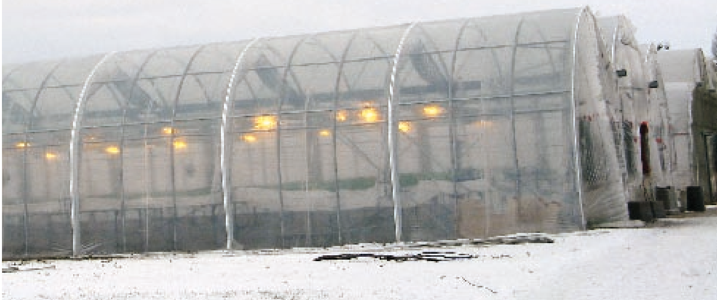
In Ontario a greenhouse with ETFE double layer inflated to benefit from the high light transmission and energy saving (picture P.A.T.I. S.p.A.).
