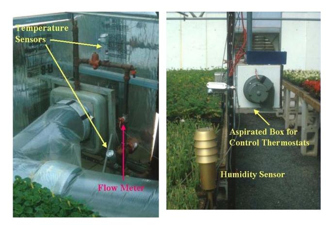
Heat exchanger, inlet/outlet temperature sensors and flow meter to determine energy input by the heat exchanger. Return to heat exchanger text
