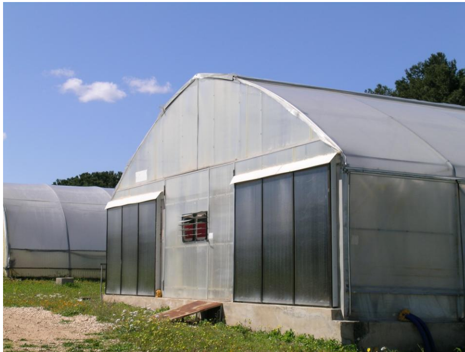
Figure 5. Solar thermal flat collectors mounted on the south-facing greenhouse surface at the experimental farm of the University of Bari, Italy.
