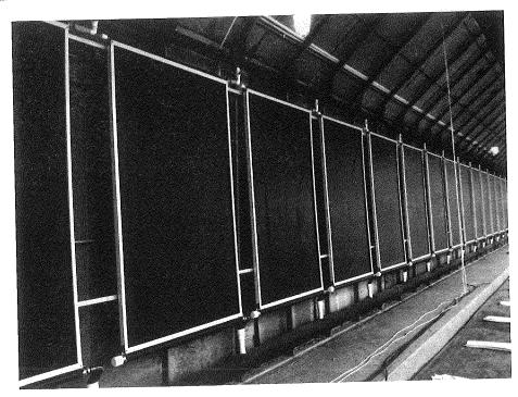
Because the back wall in the New Chinese Solar Greenhouse is not needed as a heat accumulator anymore, the wall can be made from insulating panels. These allow for an easy and rapid building of the greenhouse.
