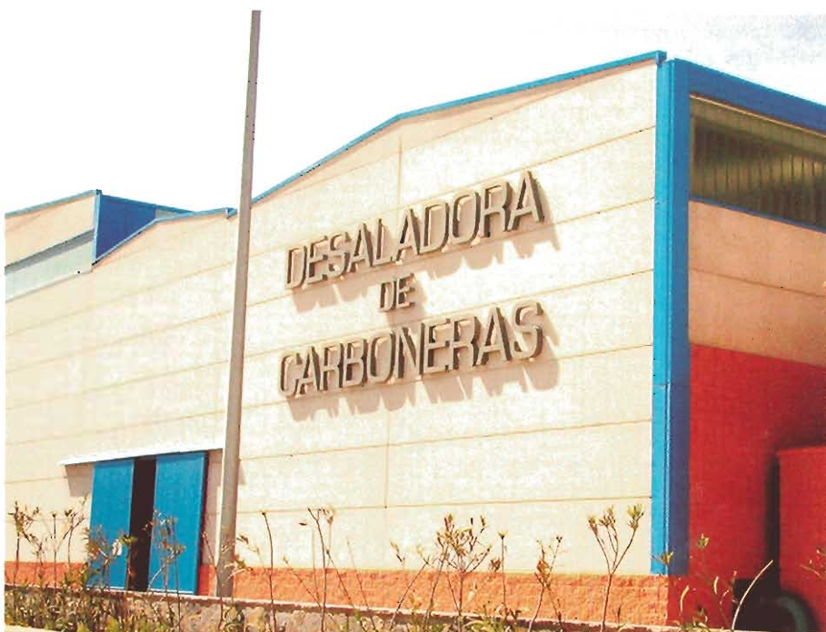
Figure 9. Seawater desalination plant in Carboneras, Almeria (Spain).
