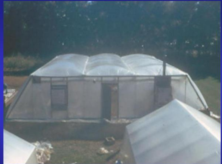
First cable supported greenhouse constructed without rafter or hoop supports
