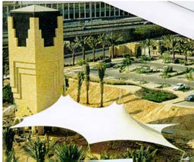
Fig. 5: The Cool Tower after construction
